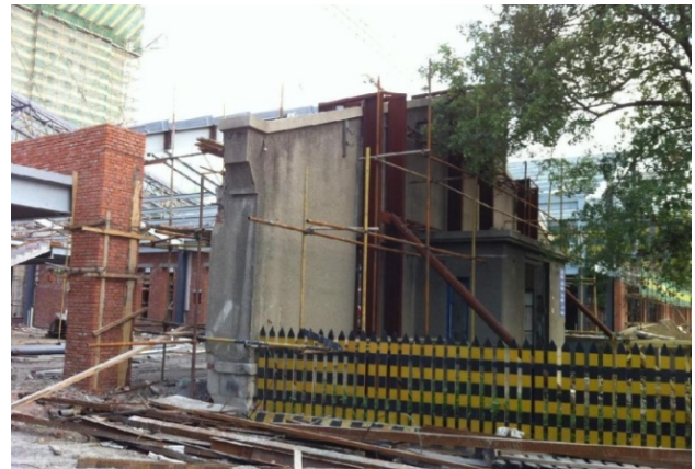
Fig. 10. Strengthening of load-bearing brick walls building of a stamping shop with a technical office (photo by Liu Fang)
