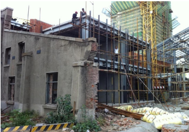
Fig. 9. Adjustable additional volume with a supporting steel frame (photo by Liu Fang)
