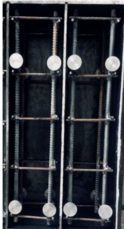
Figure 3. Reinforcement cage inserted in concreting formwork
